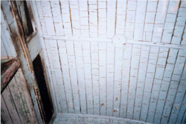
Passenger saloon ceiling showing ceiling beading and rose.
